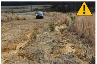
Soil is eroding from this old log deck/truck turnaround. Regrading and stabilization groundcover are needed.
