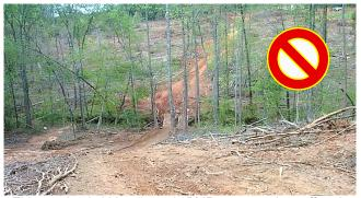
This overland skid trail needs BMPs to control runoff and minimize sedimentation into the stream.
