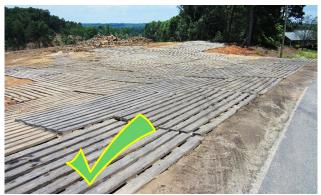
This log deck is on a recently completed job. It is on flat, stable soil. Road pallet mats provided a firm base for log trucks and minimized sedimentation onto the roadway.
