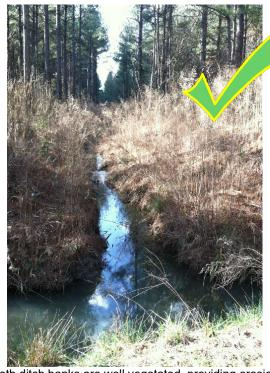
Both ditch banks are well vegetated, providing erosion and sedimentation control. The ditch corridor is open with no timber to allow maintenance access.
