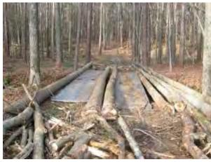
Figure 1b: A set of two bridgemats with log stringers installed for a skid trail crossing of a stream in central North Carolina.
