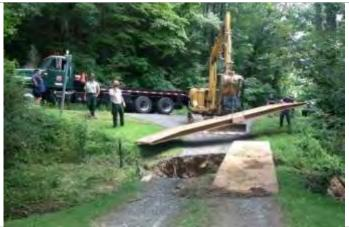
Figure 15: July 2013, NCFS Ashville District's bridgemats being installed for public road access after flooding in Madison County, NC. The bridgemats provided homeowners access to their homes until the crossing could be repaired.
