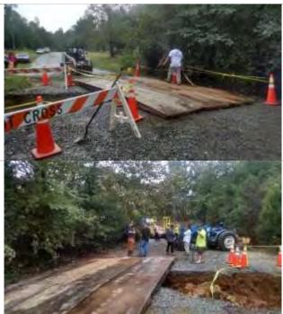
Figure 16 (above two pictures): September 2016, NCFS Hillsborough District's bridgemats installed for public road access following Hurricane Matthew in Alamance County, NC. This temporary fix provided access to dozens of homes and was highlighted by local television media.
