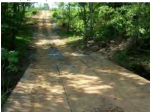
Figure 1a: A set of three bridgemats installed for a haul road crossing of a perennial stream in central North Carolina.
