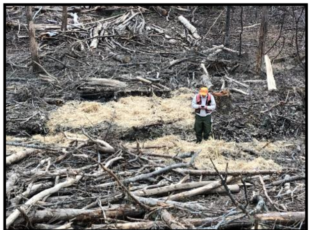
Slash and straw at a former skid trail stream crossing (above). Wood chips spread across a deck (left).
