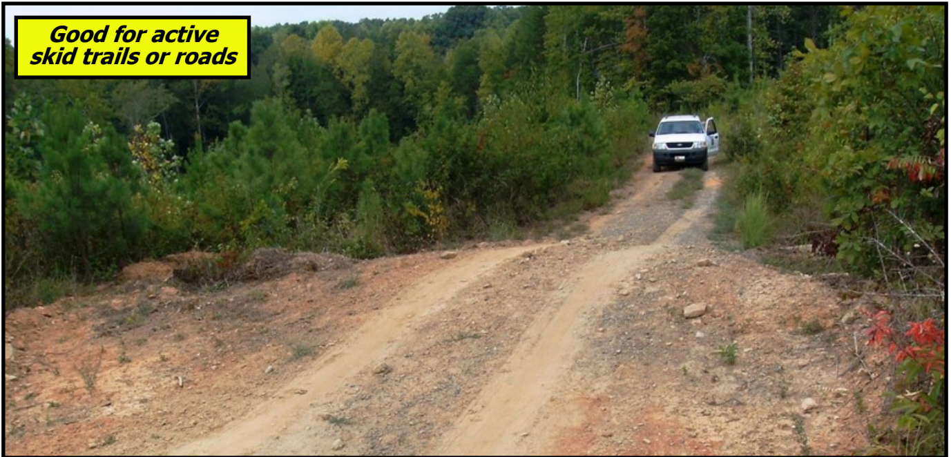
Pictured above is a rolling dip on a forest haul road. Illustrated below is an idealized schematic of a rolling dip.
