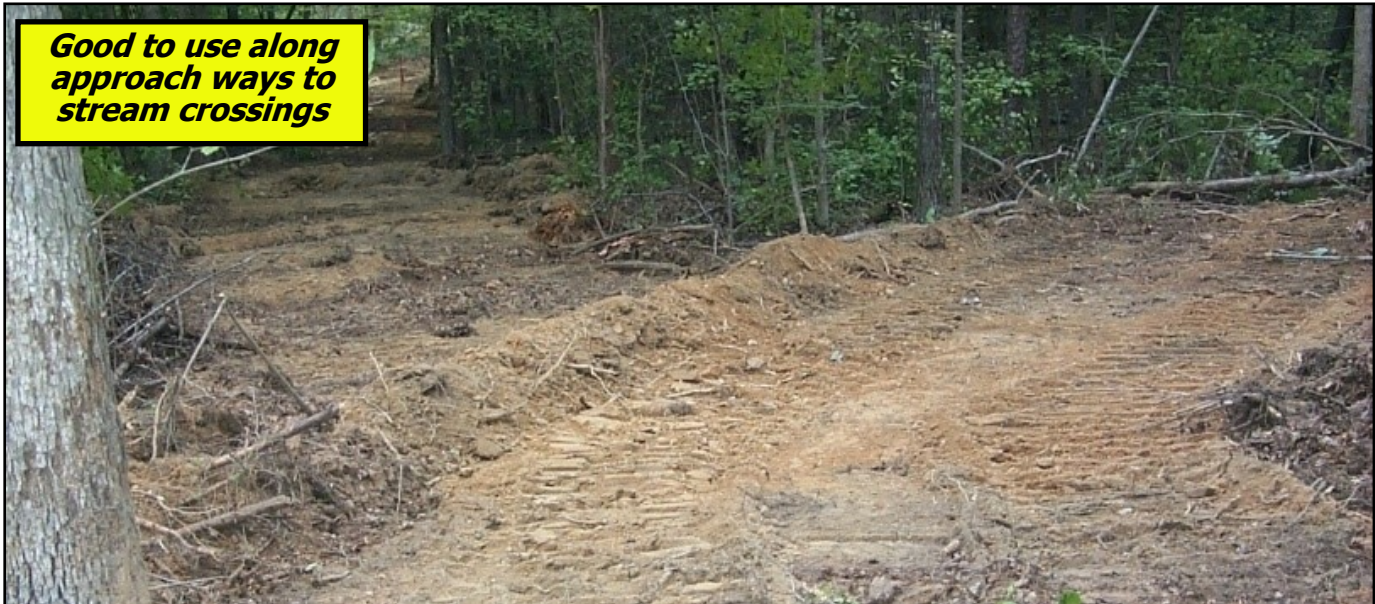
Pictured above is a turnout used together with a water bar on a skid trail.
