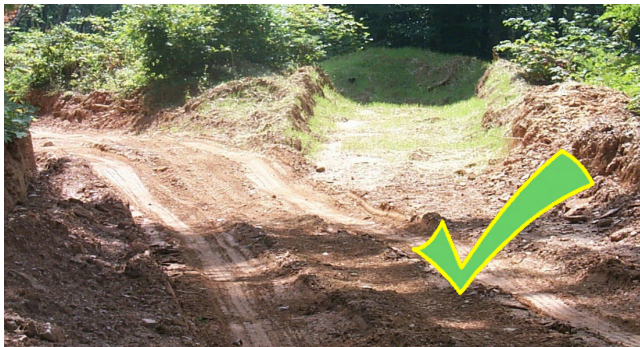
This turnout on an active logging road has grass cover.
