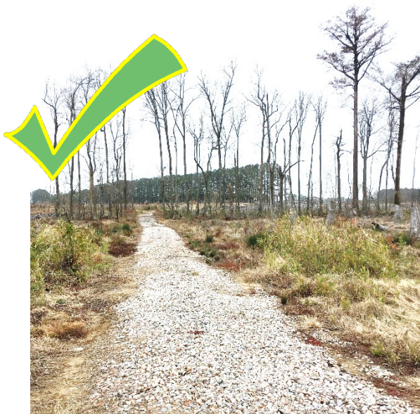
A well done wetland forest road with its overall footprint kept to a minimum. No ditches were dug.
