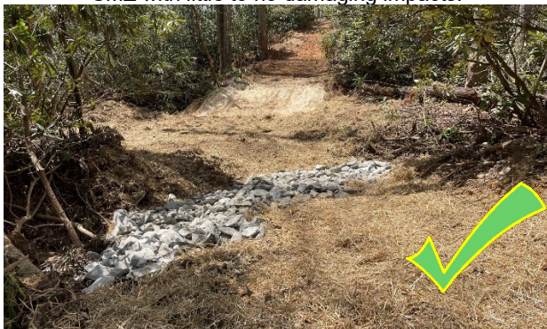
This fireline was rehabilitated and stabilized.
