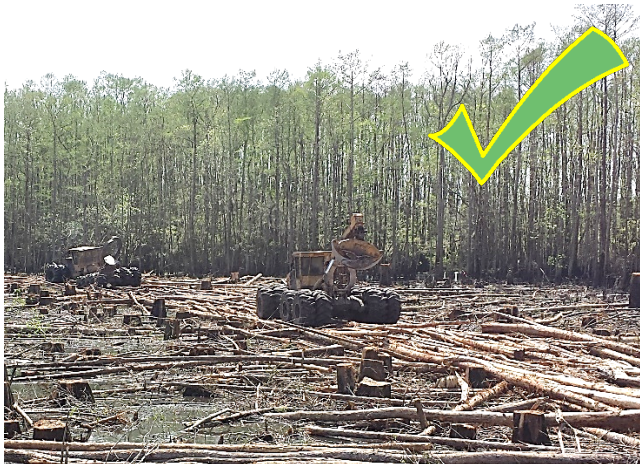
A shovel skid trail for a wetland forest timber harvest.
