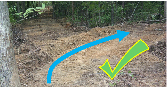
This waterbar ties into a turnout to divert runoff from this closed out skid trail.
