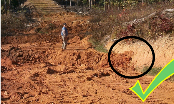
Waterbar is tied in with the cut bank slope.
