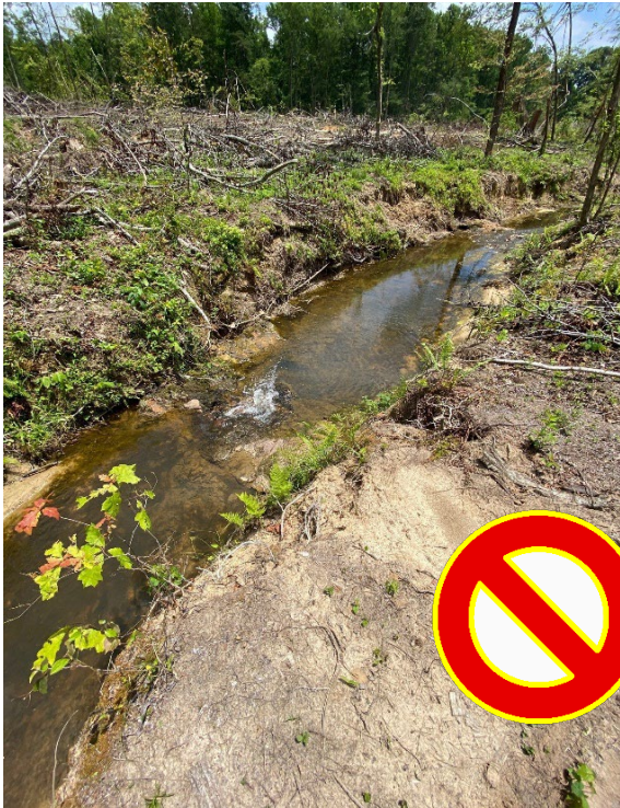
SMZ on this perennial stream was clearcut, which is a violation of the FPGs.
