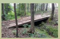
**Left:** A set of properly installed bridgemats protecting the stream channel;
