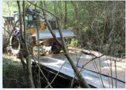
**Above:** NCFS bridgemats in use on a logging job in Halifax County. **Below:** NCFS bridgemats installed over road washout as temporary access in Alamance
