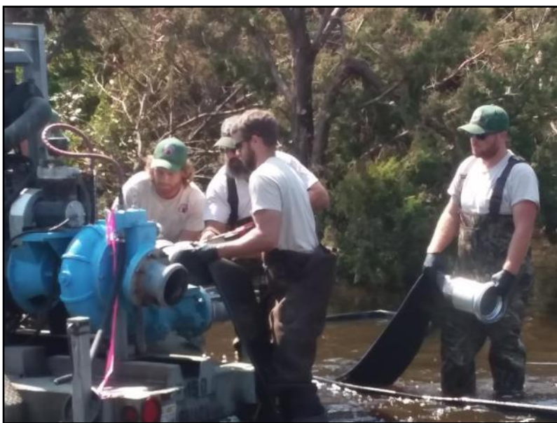
Pictured above are N.C. Forest Service personnel setting up a water pump to move floodwaters.
