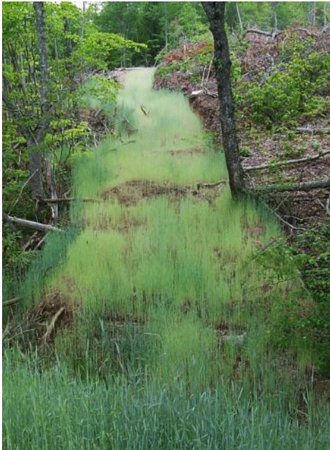
This issue's cover photo shows how well rye grass seed can germinate and thrive on a well closed out skid trail in the mountains region. Note the waterbars (earthen speed bumps) up the trail keeping runoff from becoming concentrated down the trail. Nice work!
