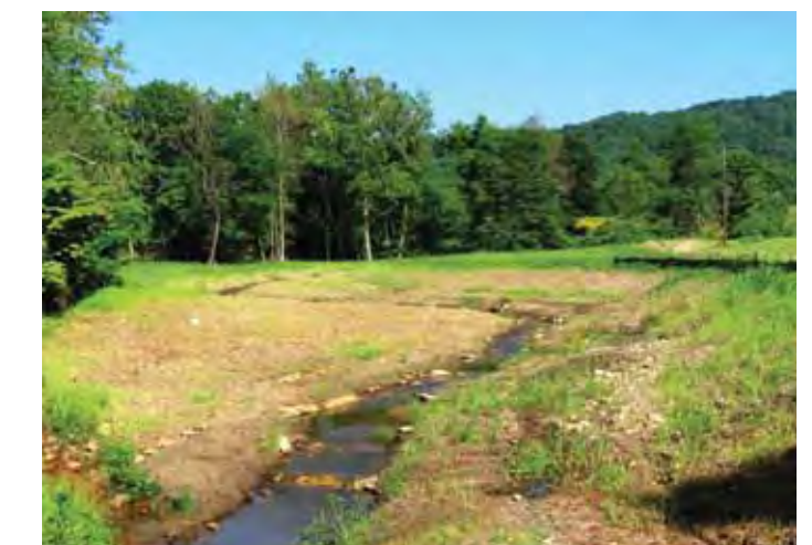
AFTER, July 2009: A new floodplain and riparian corridor was created in a former hay pasture, allowing Purlear Creek to be relocated away from the road in a natural, meandering form.
