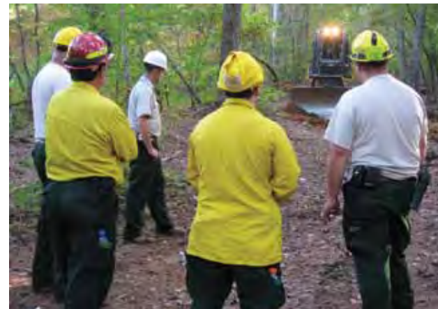
Equipment operators watch a fellow FFEO install a waterbar diversion on a trail with a DFR fire-fighting bulldozer tractor. These diversions control runoff on sloping trails and fire lines.
