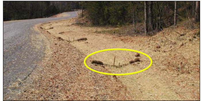
A series of coir fiber check dams (circled above) and straw matting along a gravelled road.
