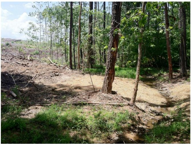
Photo 5. This stream crossing and approach way in the Piedmont ecoregion has been stabilized with straw and slash.
