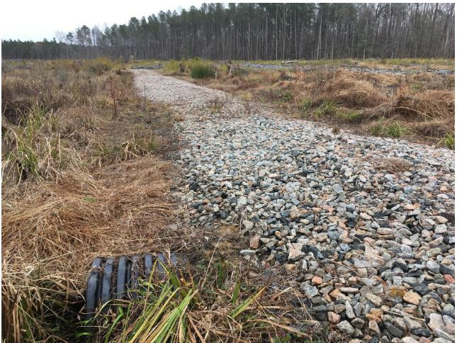
Photo 10. A well maintained minimum standard forest road on a site in the Coastal Plain ecoregion. A cross drain can be seen in the foreground allowing water to freely move through the area. Additionally, the stone surface helps to reduce erosion and rutting, while also allowing for more effective vehicle traffic in wet conditions.
