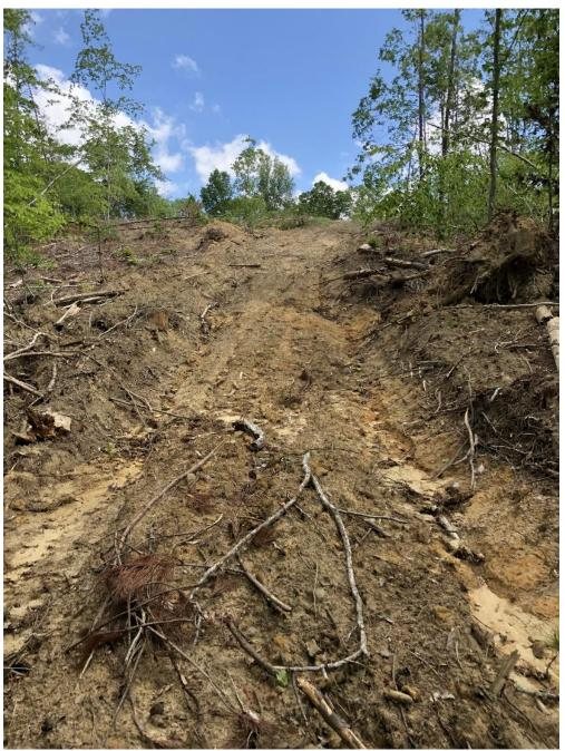
Photo 7. Erosion could be lessened along this long and steep sloping skid trail in the Mountain ecoregion by installing waterbars and turnouts to divert runoff in smaller increments onto more stable ground.
