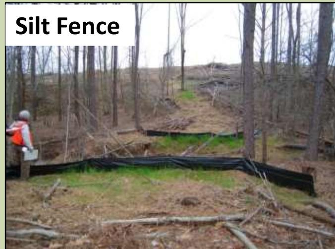
Waterbars, fescue, lime, fertilizer, straw mulch, & silt fence at the stream
