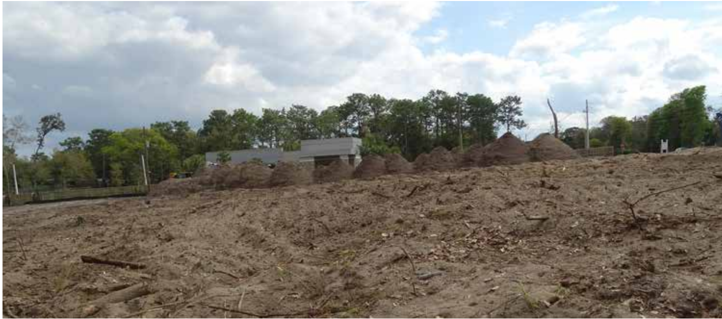
Clearing an entire site before building destroys the site's natural beauty and removes nourishing topsoil.
