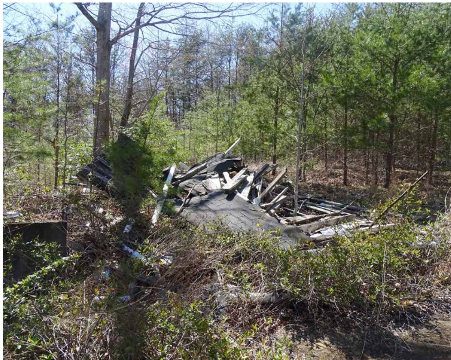
Remains of a structure found on a site that require removal.
