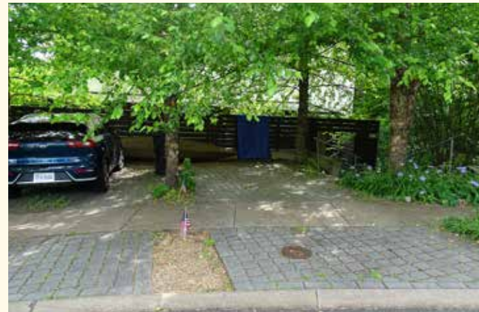
Permeable parking in a residential subdivision.
