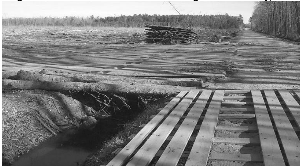
Figure 4F: Stabilized roadside ditch crossing in Bertie County, N.C.
