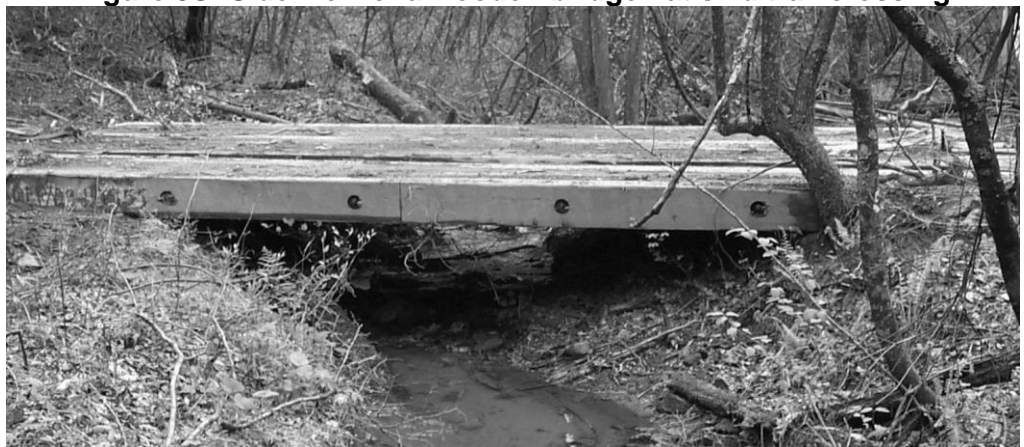
Figure 5S: Side view of a wooden bridgemat skid trail crossing
