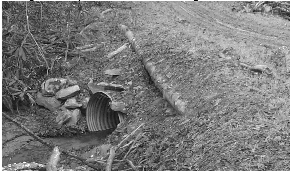
Figure 5Q: A permanent stream crossing on a forest road
