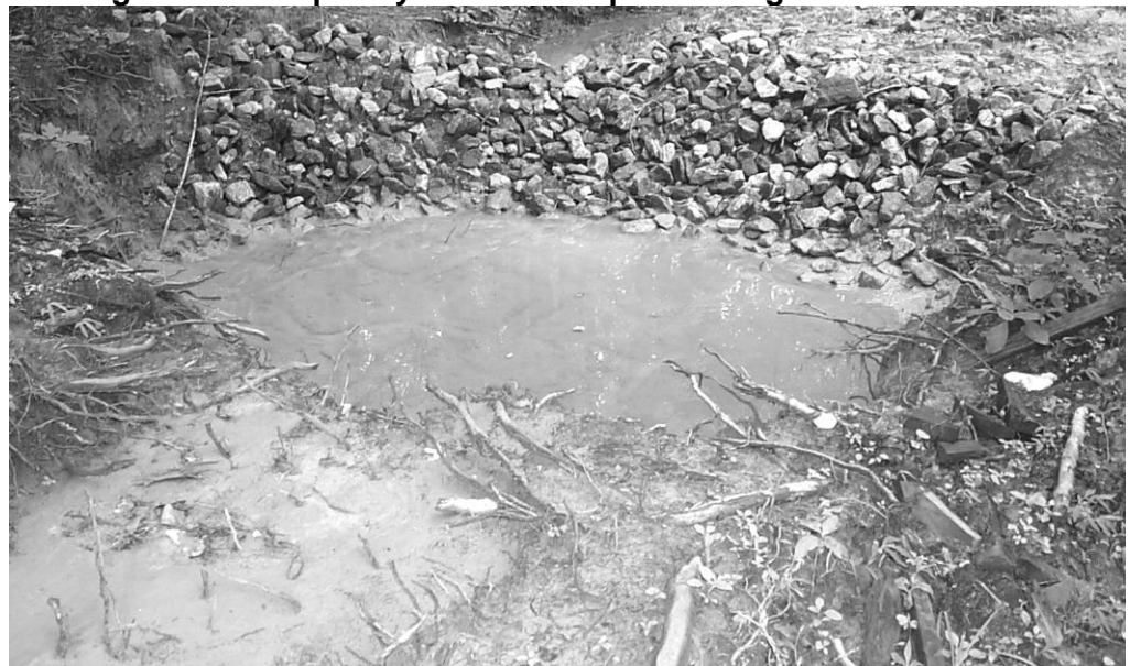
Figure 5J: Temporary sediment capture alongside a forest road
