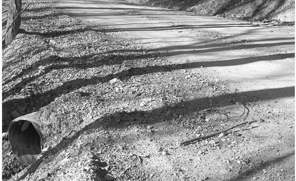
Figure 5H: View of the outlet end of a cross-drain installed underneath a permanent forest road in Wilkes County, N.C.
