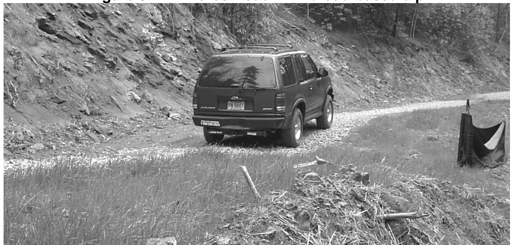
Figure 5AA: A forest road with broad-based dip
