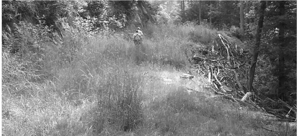
Figure 5N: A brush barrier alongside a closed road in Caldwell Co., N.C.
