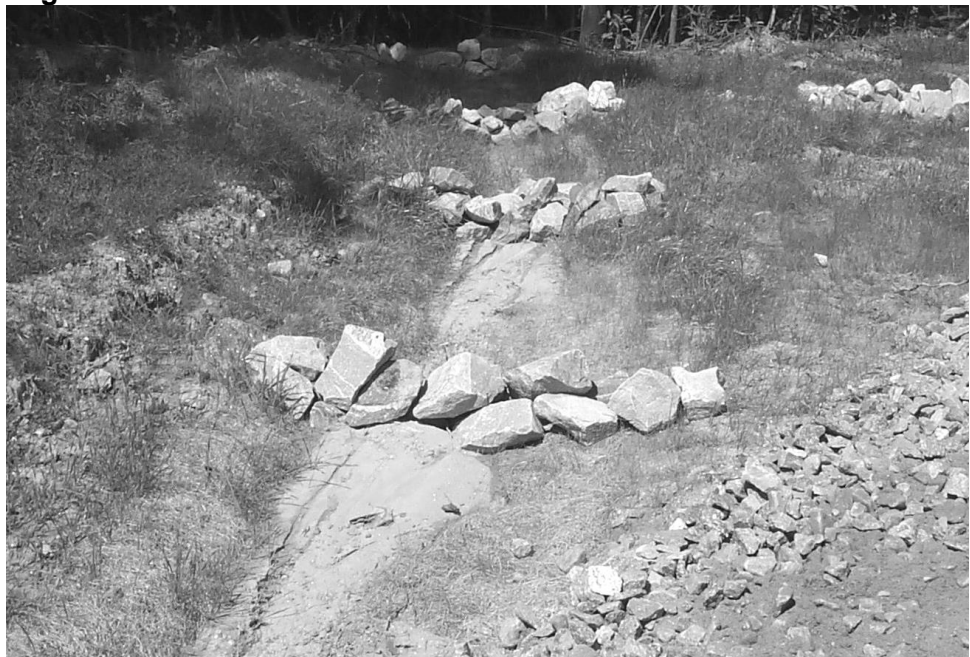
Figure 5P: Check dams installed within a turnout from a forest road
