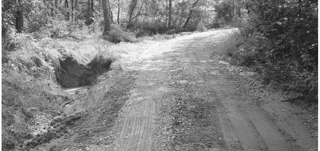
Figure 5K: A functioning sediment pit excavated alongside a forest road
