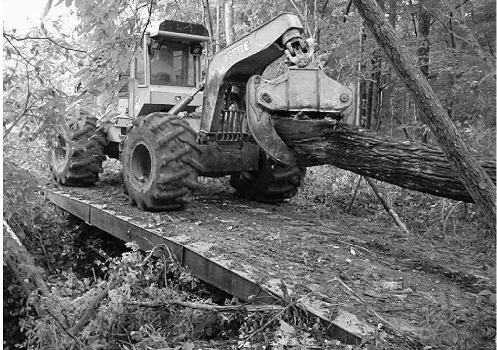
Figure 5T: Steel bridgemat installed for a skid trail stream crossing
