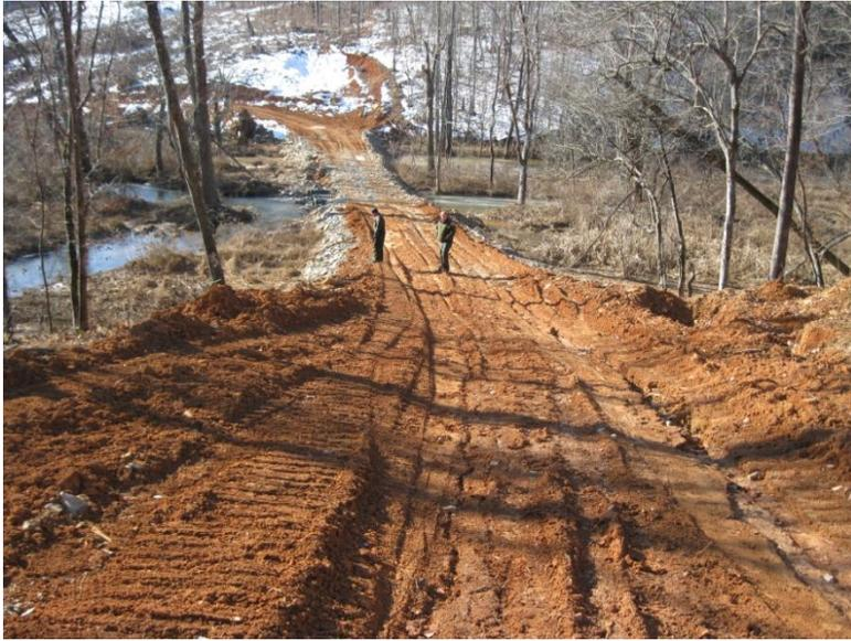
*Gravel is starting to get pushed down into the soft soil. Ruts are forming near the bridged stream crossing. Applying more gravel and/or re-grading will help.*
