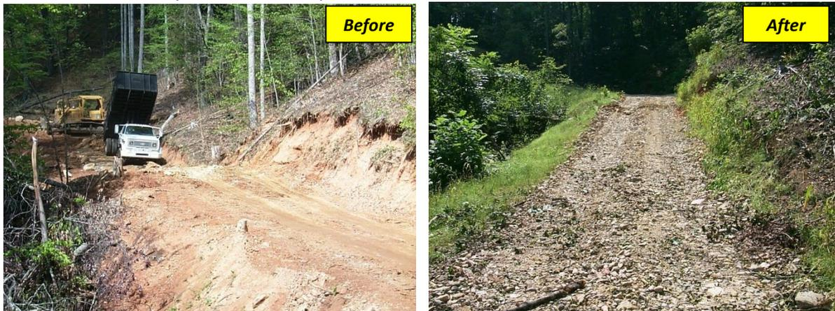
*Left: A new road being constructed. Right: Same road, after gravel surfacing and groundcover vegetation was applied. Remember: A good appearance leads to good perceptions, and an ugly appearance will leave a long lasting bad impression with the neighbors.*
