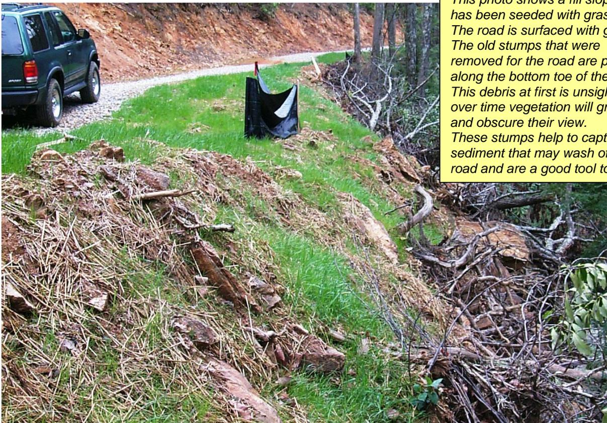
*This photo shows a fill slope that has been seeded with grass. The road is surfaced with gravel. The old stumps that were removed for the road are piled along the bottom toe of the slope. This debris at first is unsightly, but over time vegetation will grow up and obscure their view. These stumps help to capture any sediment that may wash off the road and are a good tool to use.*
