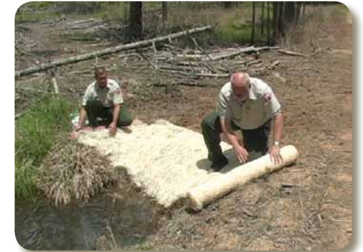
Two screen-shots from the video, showing silt fence installation (left) and erosion control matting (right).
