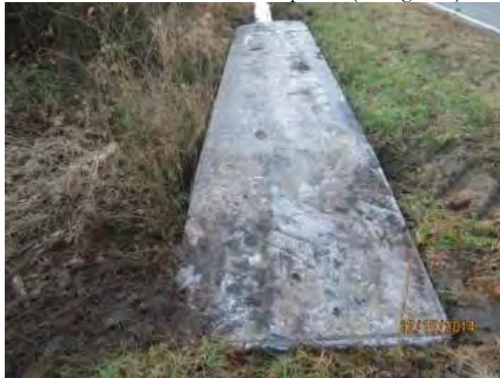
*Figure 3. NCFS bridgemats used in Edgecombe County, 2014 to protect a ditch from sedimentation.*
