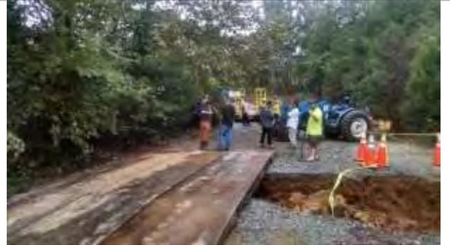
Figure 16 (above two pictures): September 2016, NCFS Hillsborough District's bridgemats installed for public road access following Hurricane Matthew in Alamance County, NC. This temporary fix provided access to dozens of homes and was highlighted by local television media.
