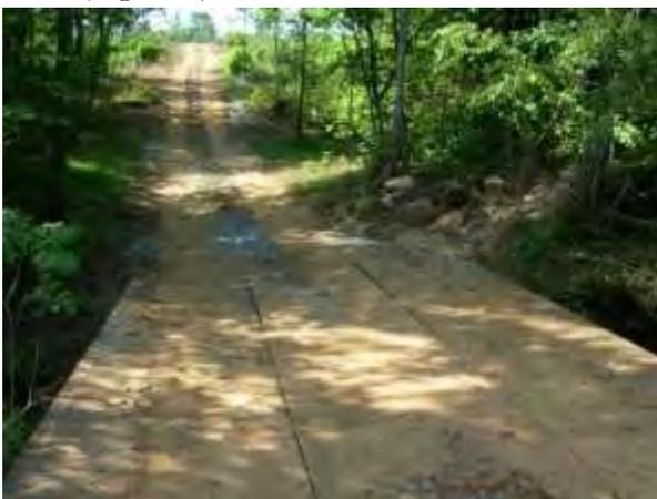
Figure 1a: A set of three bridgemats installed for a haul road crossing of a perennial stream in central North Carolina.
