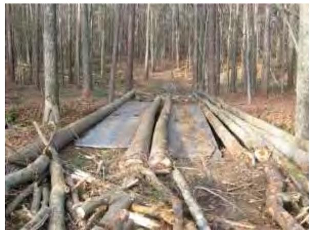
Figure 1b: A set of two bridgemats with log stringers installed for a skid trail crossing of a stream in central North Carolina.
