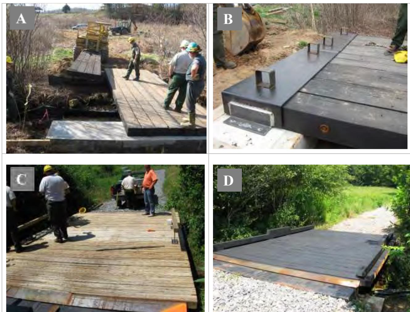
Figure 11. A) Installation of treated **Emtek™** wooden bridgemat panels over Purlear Creek, B) Metal end-cap securing wooden panels to the concrete abutment, C) Cross decking installed atop the initial bridgemat paneling. D) Completed installation of the demonstration bridge.
