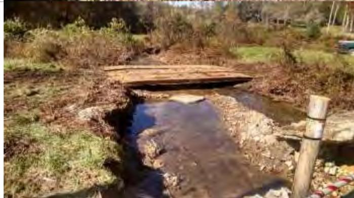
Figure 17 (left two pictures): November 2017, NCFS Asheville District's bridgemats were installed following severe storms caused damage to a low-water crossing in Buncombe County, NC. NCFS Bridgemats were placed about 30-ft upstream and served as the primary access to several homes until the crossing was repaired.
