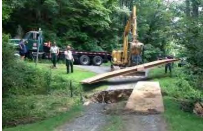
Figure 15: July 2013, NCFS Asheville District's bridgemats being installed for public road access after flooding in Madison County, NC. The bridgemats provided homeowners access to their homes until the crossing could be repaired.
