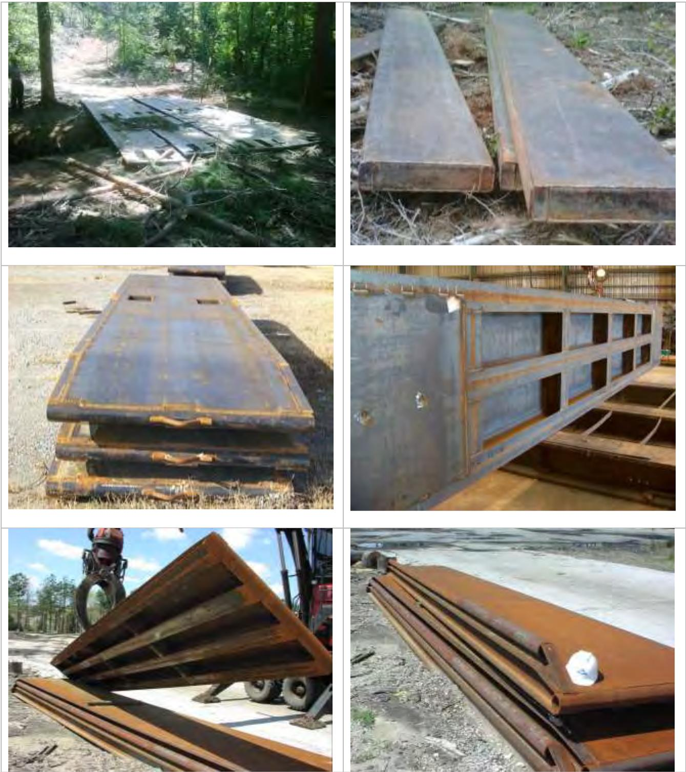
Figure 4: Six different steel bridgemat design configurations observed by NCFS staff.
