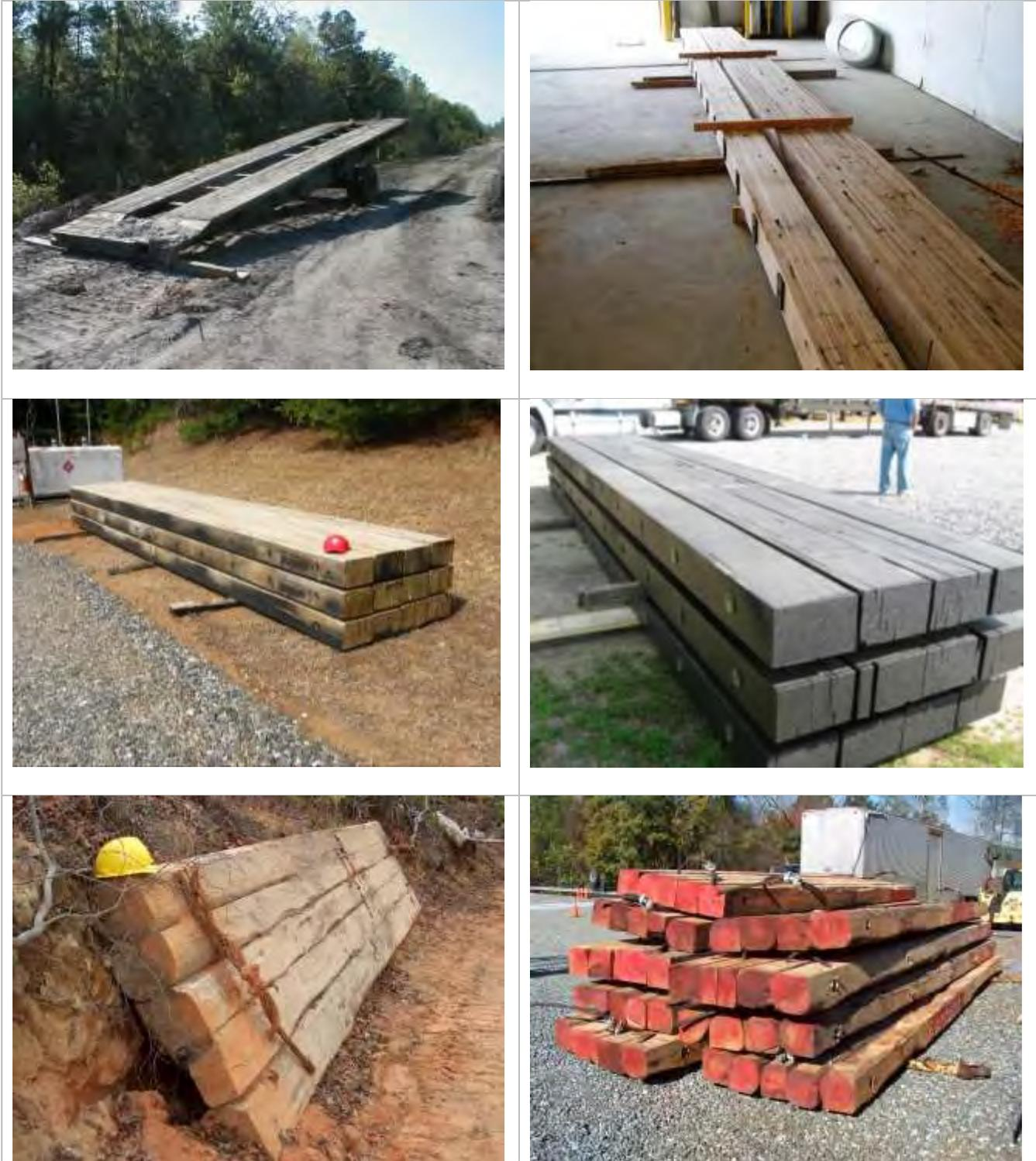
Figure 5: One steel trailer with wooden travel surface and five different wood bridemat designs/configurations.
