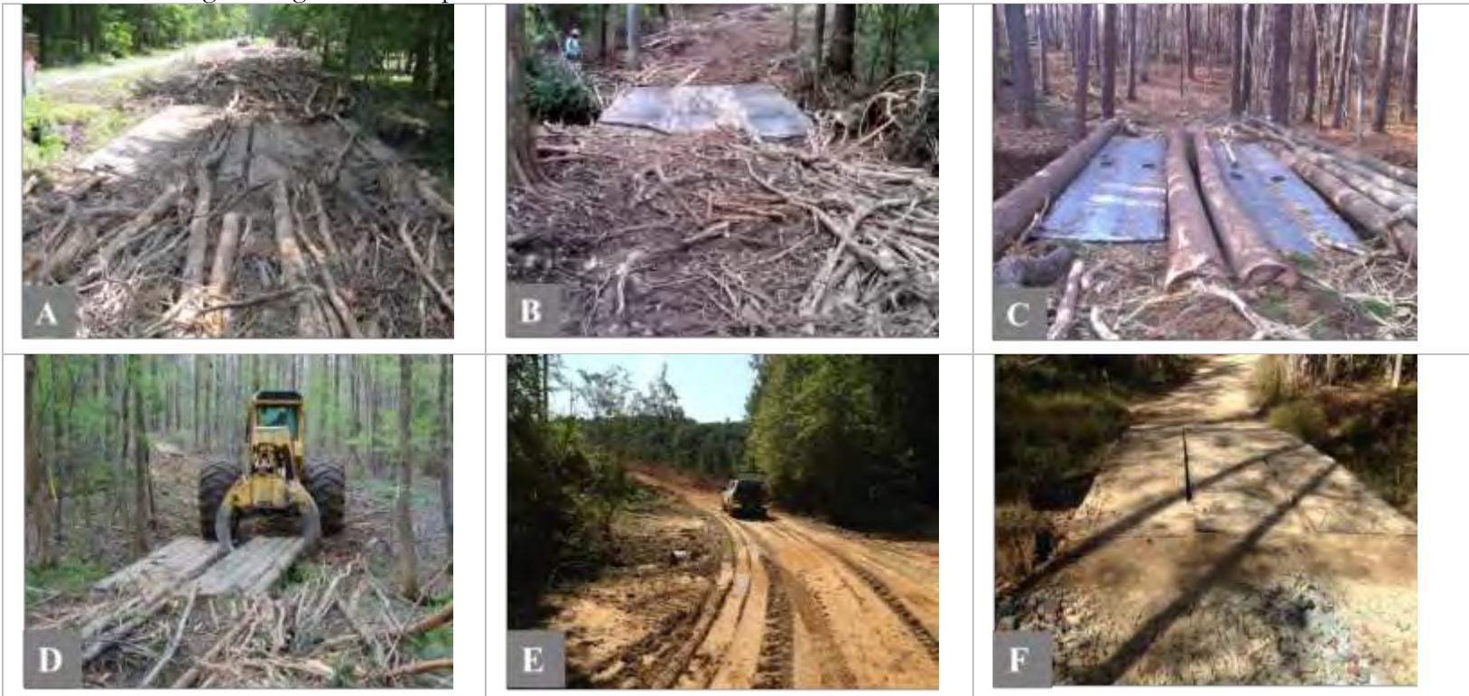
Figure 10. Stream crossing sites during forest operations as published in Boggs and others (2017). A) Wood bridgemats on temporary skid trail, B) Steel bridgemats on a temporary skid trail, C) Steel bridgemats on a temporary skid trail, D) Wood bridgemats on temporary skid trail, E) 30-inch diameter culvert on a permanent haul road, and F) Steel bridgemats on a permanent haul road.
