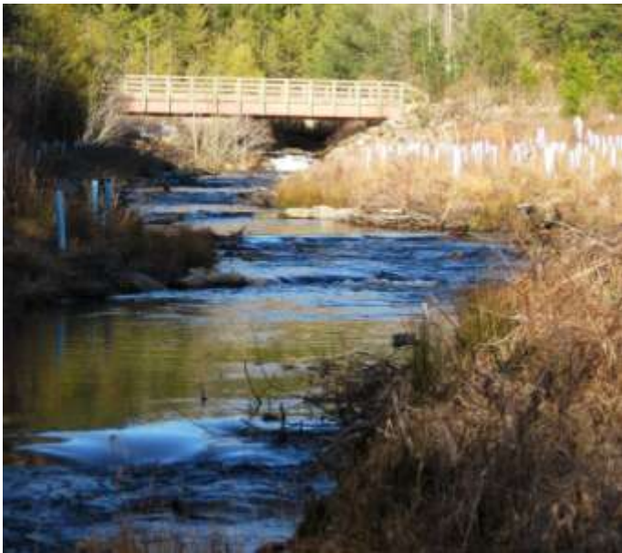
Photo Above, February 2013: View looking upstream from near the end of the restoration project.
