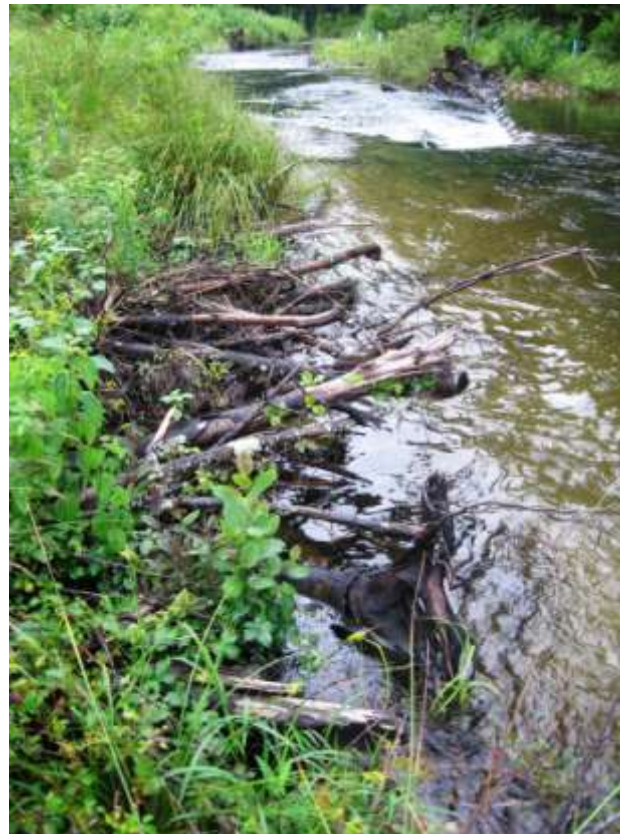
Photo Right, July 2013: Brush toe material on left bank remains intact and functioning, seen here at bankfull, or near bankfull.
