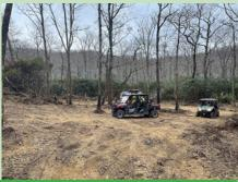
Poplar Drive - Identifying sites for water bars using the "eye level" method during the incident in an area without active fire (left). Estimating area of bare soil within a safety zone to plan for post-incident soil stabilization (right).
