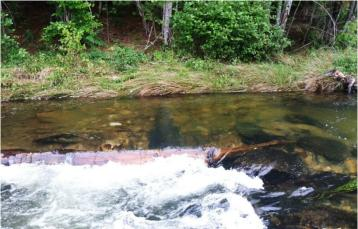
Photo from August 2013 showing a combination rock/log vane structure functioning. Note the matted down vegetation on the far bank, indicating the extent of floodplain flow.
