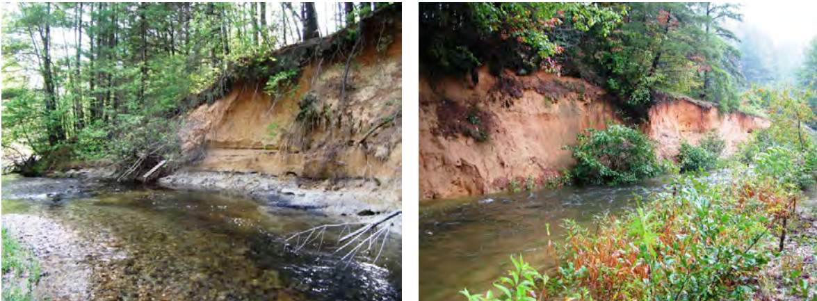
Figure 1. Reasonover Creek prior to restoration.
