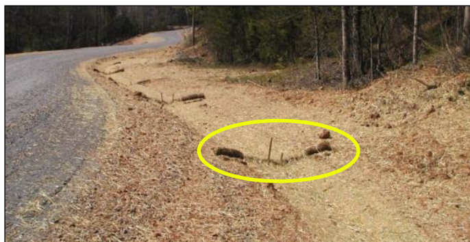
A series of coir fiber check dams (circled above) and straw matting along a gravelled road.
